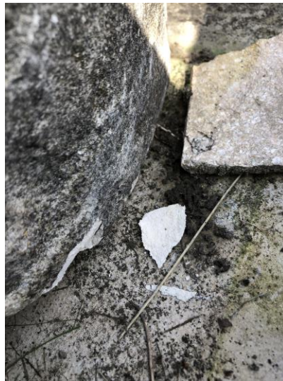
Examples of stone features having experienced material loss (left), surface flaking/chipping (middle) and stone splitting (right). Images taken by author with kind permission from Burwell Museum & Windmill .
